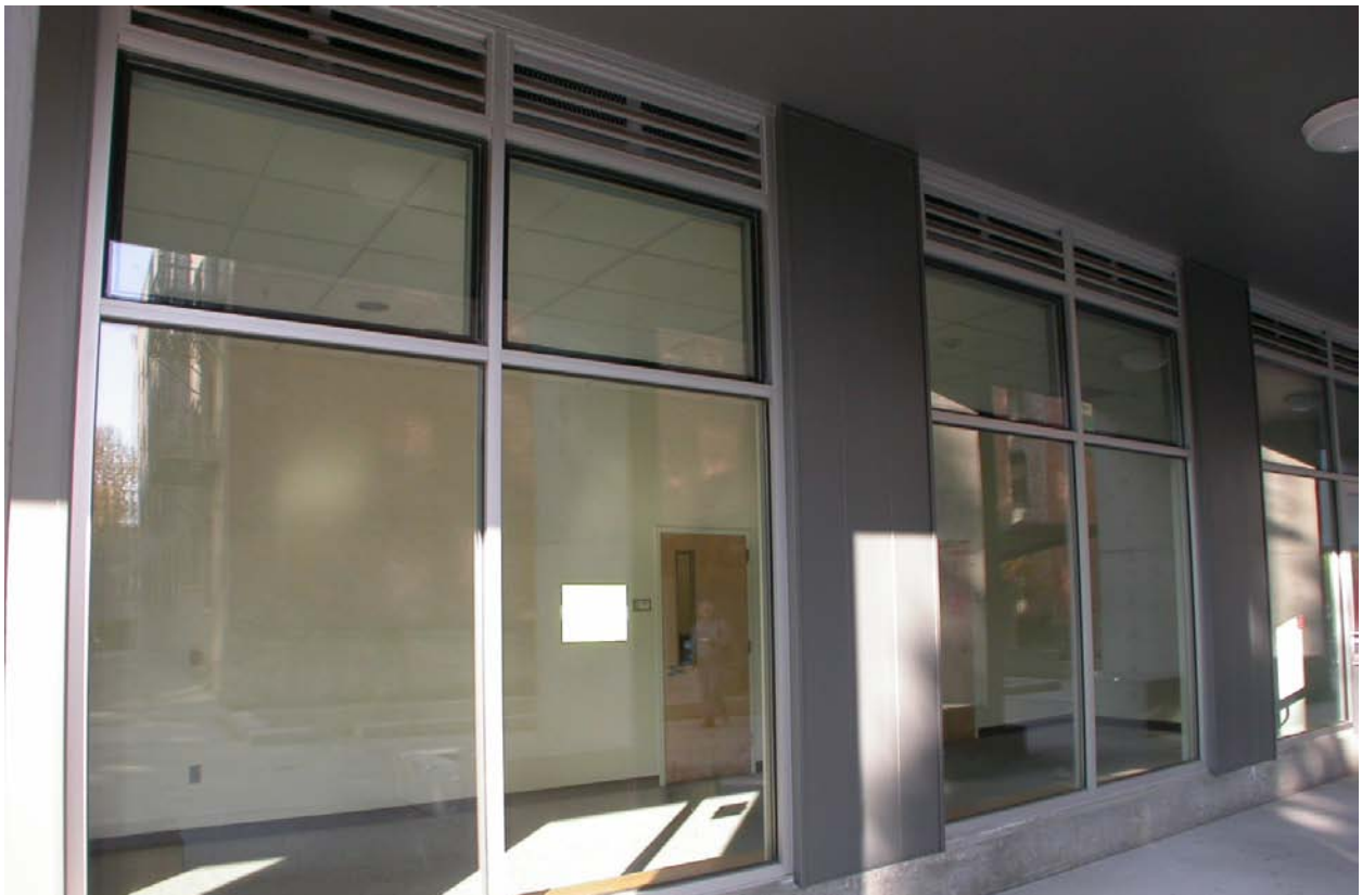
Fig. 9 Entrance hall for the ground floor classrooms
