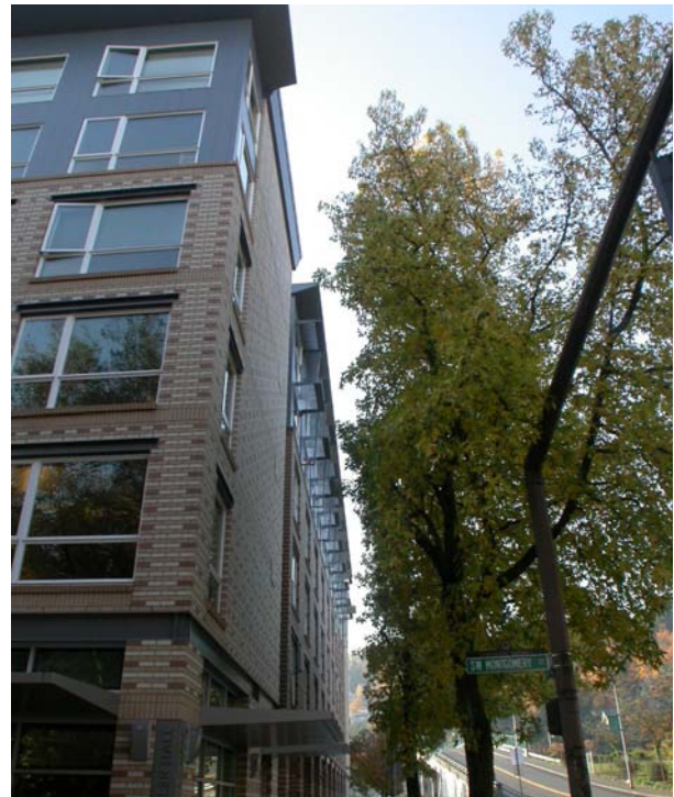
Fig. 3. Epler Hall exterior
