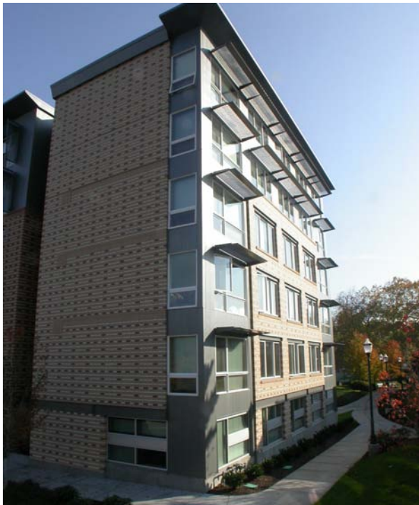
Fig. 2. Epler Hall exterior
