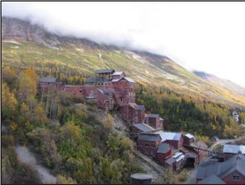
Mill Building, Kennecott Mines NHL, 2005. NPS Collection
