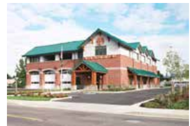
Exterior at Entrance
