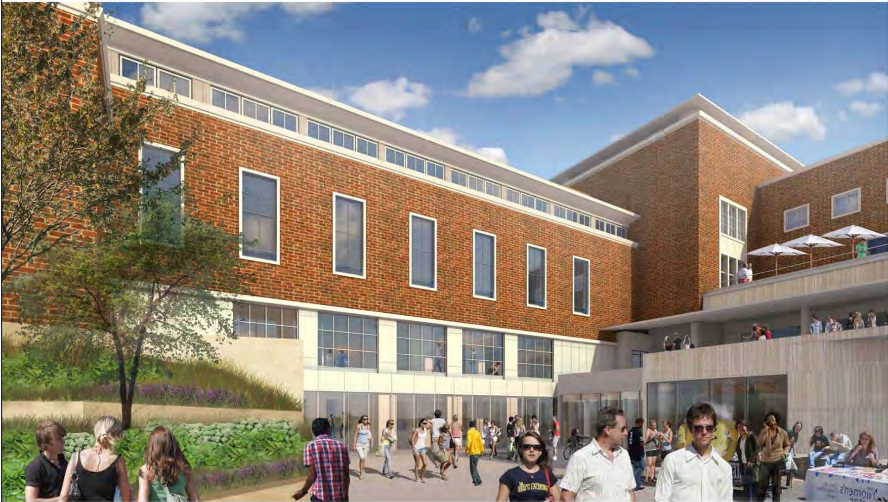
NORTHWEST MAIN ENTRY
