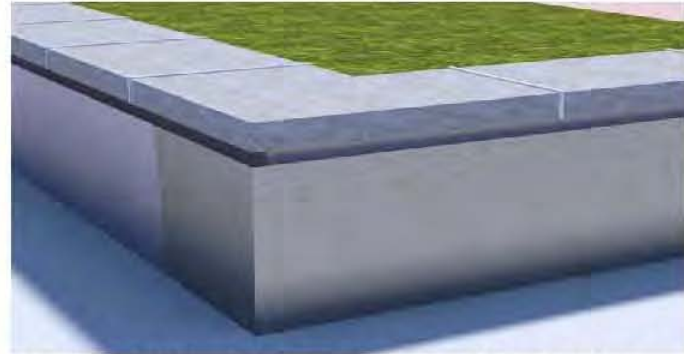
SEAT WALL WITH PRECAST CAP & SKATE STOP
