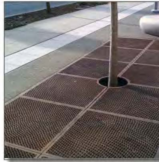
TREE GRATES & TRENCH DRAIN
