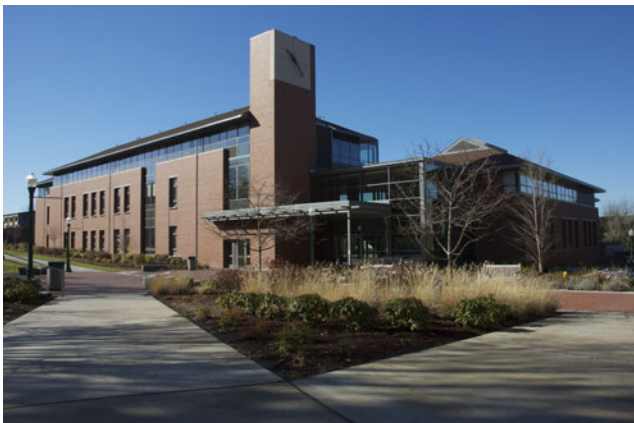
Fig. 4: Exterior view of atrium with brick tower
