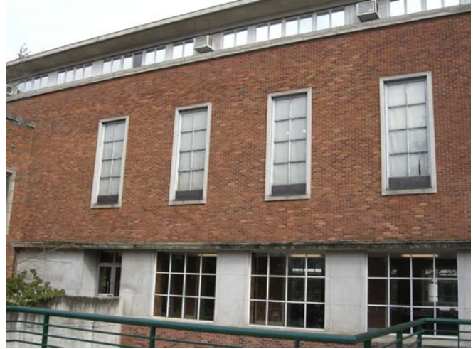
Fig. 15 Exterior shading devices may be able to improve the thermal performance of the McMillan gallery.
