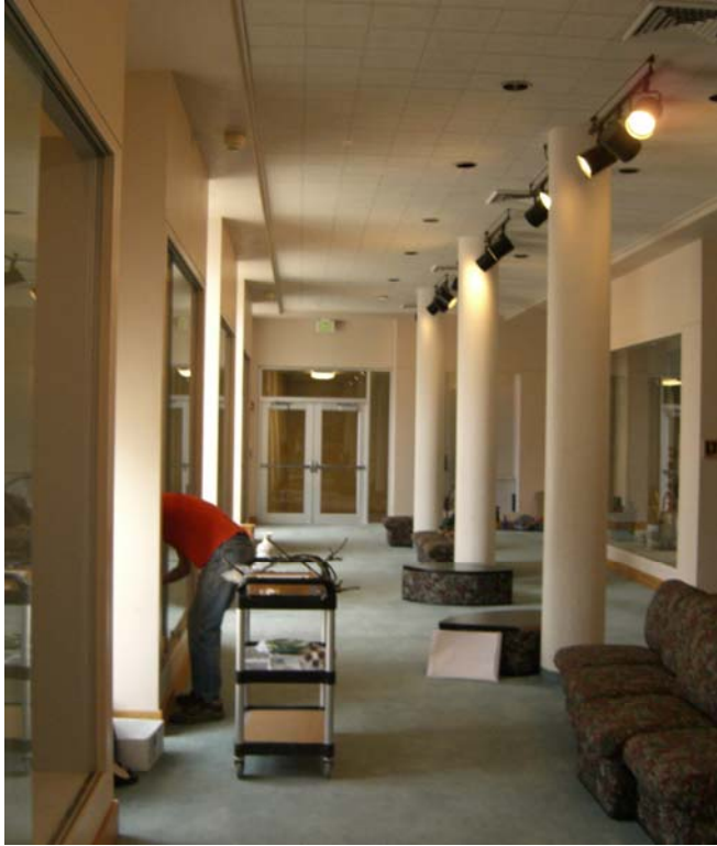
Fig. 2 A view down the warmer west side of the gallery, beneath which the room's radiant heating system is located.
