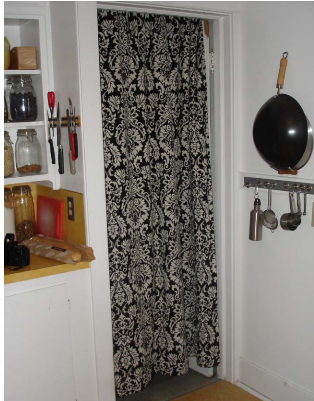
Figure 4: Curtain separating heated space from uninsulated basement
