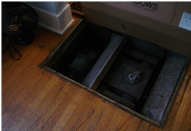
Figure 3: Vent to oil furnace
