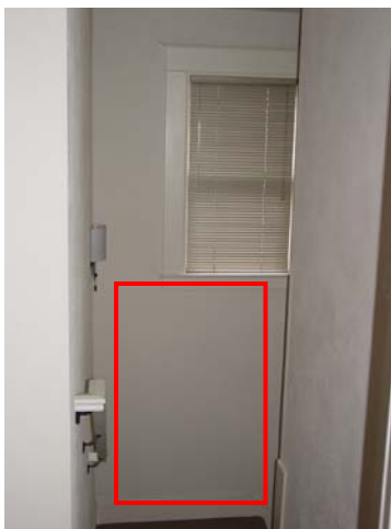
Fig. 2: Second Floor Stair Landing East Wall-1
