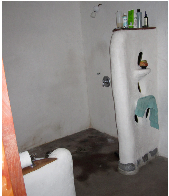
Fig. 2: Bathroom with polymer sealed walls
