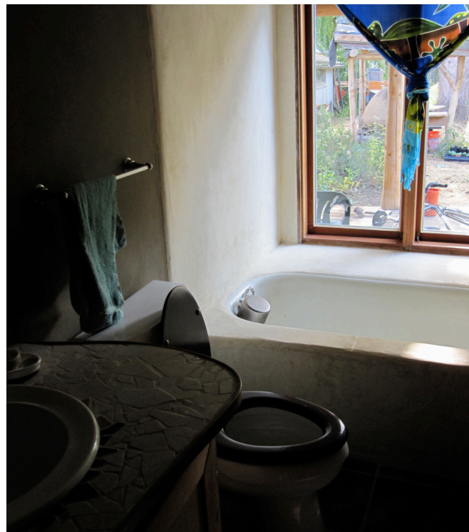
Fig. 3: Bathroom with Olive Oil Soap sealed walls
