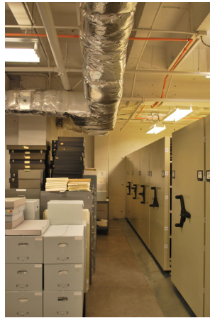
Fig. 7: ZONE 3 - back storage room
