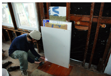
9. Install new 1/2" gypsum board to new stud wall
