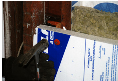
6. Fasten Rigid Foam EPS Insulation to studs
