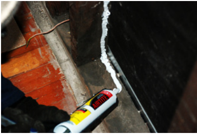
1. Caulk to existing framing
