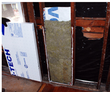
5. Caulk studs for 2" Rigid Foam EPS
