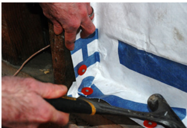
3. Fasten Tyvek to studs
