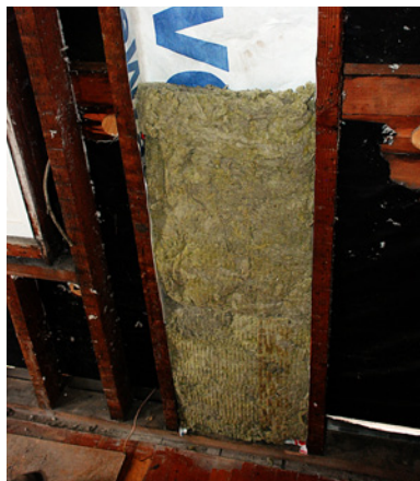
4. Fill with R-15 Rockwool Batt Insulation
