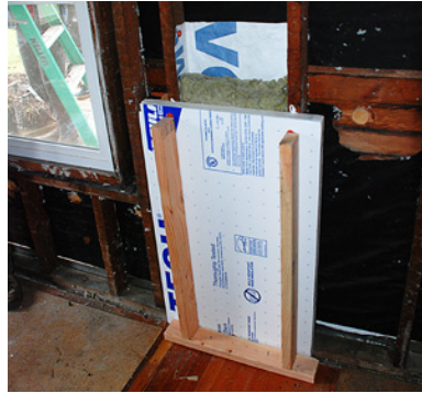
7. Install New 2x4 stud wall against EPS
