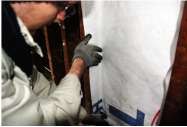
2. Embed Tyvek in caulk for each bay
