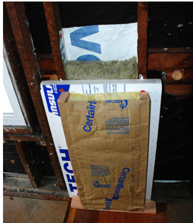
8. Install R-15 Kraft-faced fiberglass batt insulation
