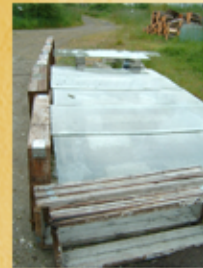
3. The Drying Kiln: The forms can be removed from the blocks in about one hour. Reused glass panels are then supported on concrete blocks to protect the papercrete from moisture and expedite the curing process.
