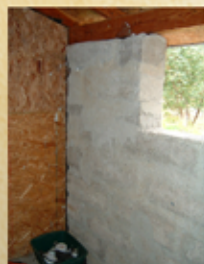
An addition to a house using papercrete as infill within post-and-beam construction. The infill consists of blocks and mortar bound with layers of papercrete stucco.
