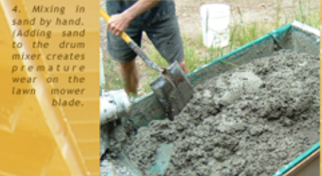
4. Mixing in sand by hand. (Adding sand to the drum mixer creates premature wear on the lawn mower blade.)
