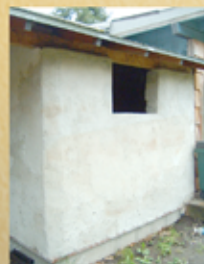
An addition to a house using papercrete as infill within post-and-beam construction. The infill consists of blocks and mortar bound with layers of papercrete stucco.
