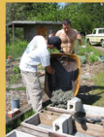
1. The finished papercrete mix is transferred into reusable forms made from scrapwood.
