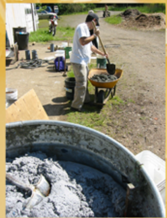
4. Mixing in sand by hand. (Adding sand to the drum mixer creates premature wear on the lawn mower blade.)
