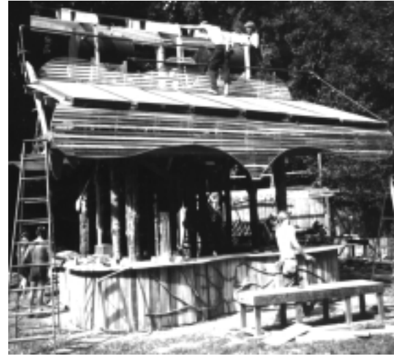
"Solar Bozos" work on Energy Park's new Information Booth, July 1995.
