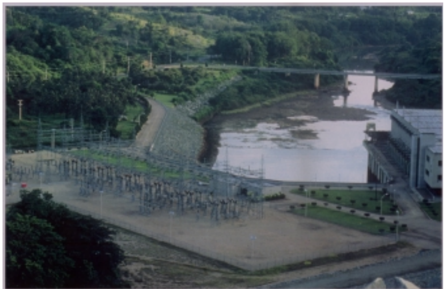
Sirikit Dam, one of the two major providers and controllers of water supply in the Central Plain of Thailand. Photo by M.L. Thosawan Dhevakul.
