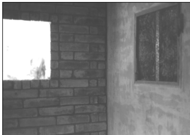
Cache block and straw bale walls, Austin, TX.
