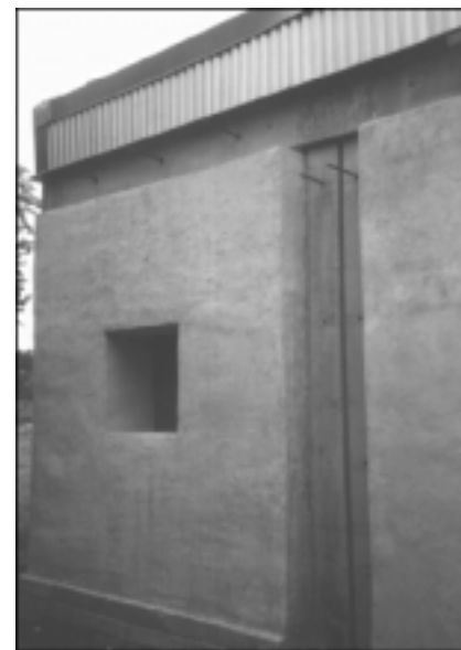
Exterior of straw bale wall, Austin, TX.
