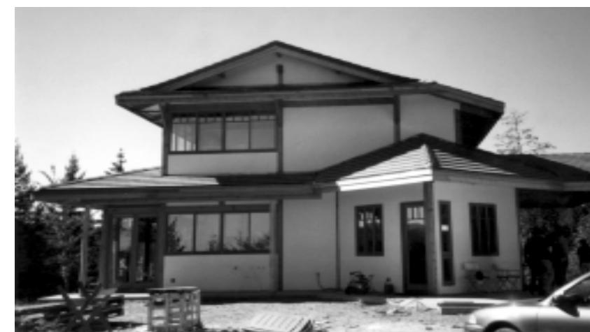
Tim's house features exposed heavy-timber construction
