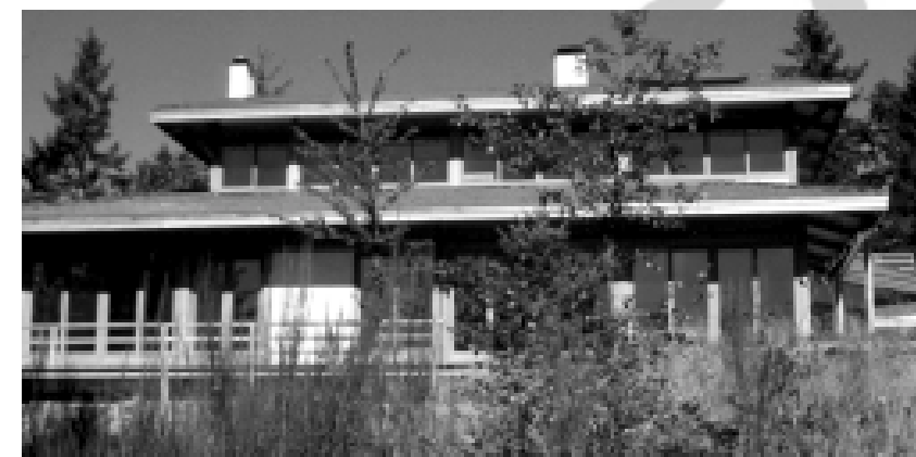
south-facing windows of the Leonard residence
