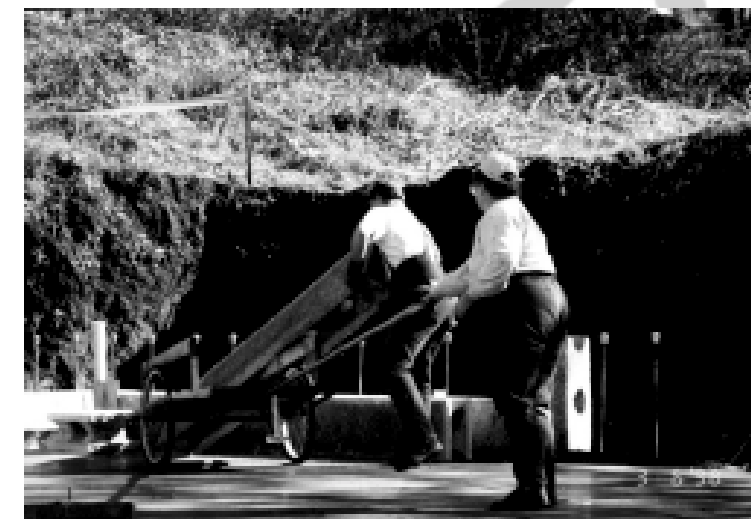
laying Rastra courses in the building of the Brule/Black residence
