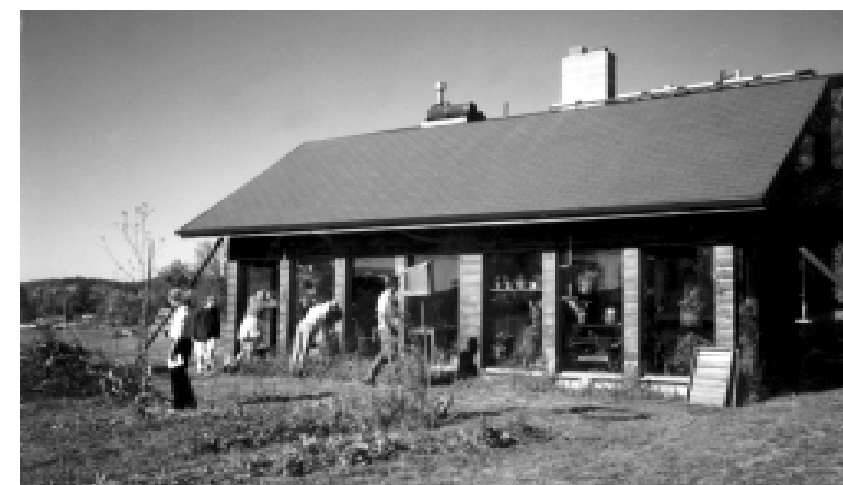
Frank Citaldo's residence features large, south-facing windows to gather the sun's heat
