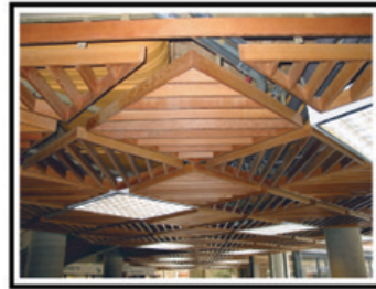
Ceiling panel detail from skylight lounge
