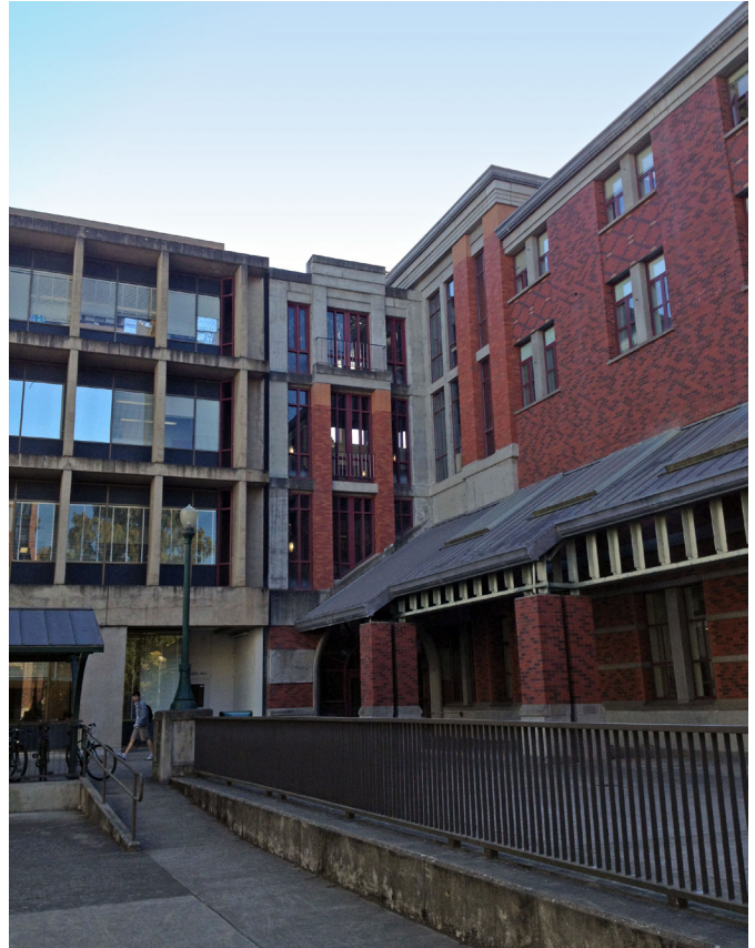
Southwest corner of Plaza as seen from courtyard
