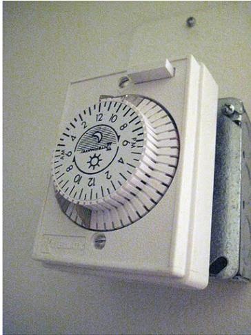
Fig. 3: The bathroom fan timer control
