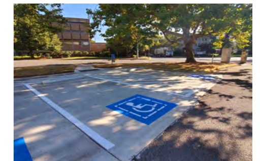
After: The same space after repairs
