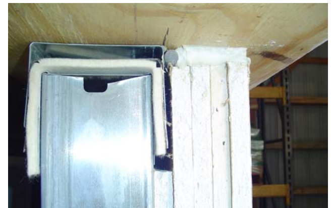
Isolated gypsum board assembly
