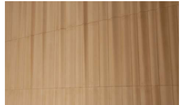
Medium scale diffusion – cast plaster panels
