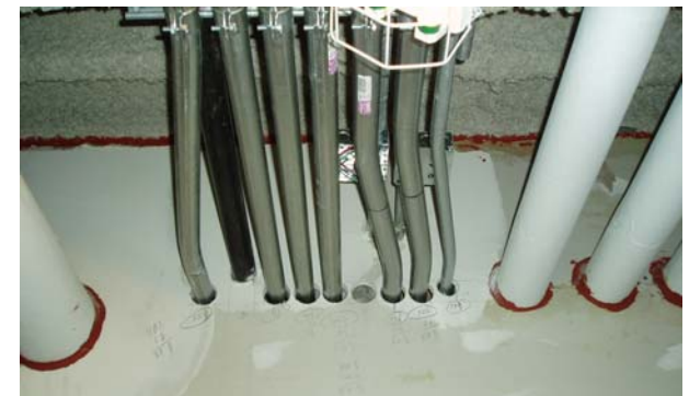
Resiliently sealed conduit and pipe penetrations
