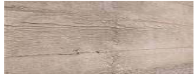
Fine scale diffusion – board formed concrete
