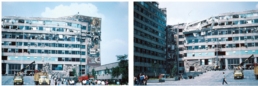
Figure 5. Photos of the damaged Secretaria de Comunicaciones y Transportes (SCT, Ministry of Telecommunications and Transportation) building after the 1985 earthquake. It was severely damaged with several collapsed floors (see USGS Photographic Library website in Data and Resources ).
