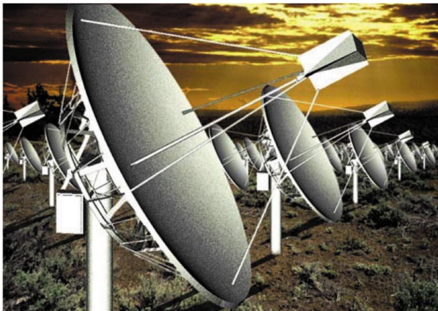
Figure 5 Artist's concept of the Allen Telescope Array at Hat Creek Observatory. 1000 3 m or 500 5 m dishes will be arrayed together to produce a radio telescope whose collecting area is 10^4 \text{ m}^2 . The array should become operational in 2005, and will be constructed from emerging telecommunications and other consumer technologies in order to keep the price as low as possible. Because the array will be able to form multiple beams within a large primary field of view, with an instantaneous frequency range of 0.5 to 11 GHz, it will be possible to do SETI and more traditional radio astronomy continuously and simultaneously. Recent design reviews have concluded that the most cost effective antennas for the ATA will be 350 6.1 meter offset Gregorian reflectors with 2.4 meter secondaries and a ground shield. The current design concept can be seen at http://www.seti.org/science/ata.html
